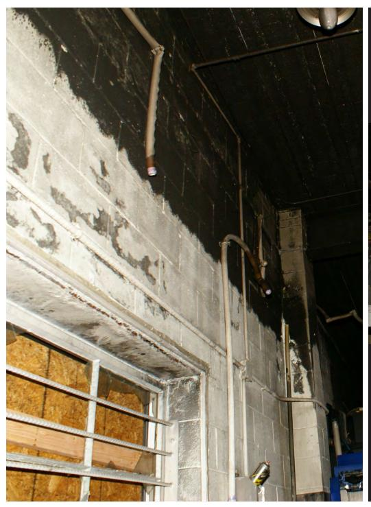
No surface was untouched from the ceiling to the floor. Intense scorch marks, dark soot and extensive heat damage devastated the shop. Note the intense and visually graphic heatline around the perimeter of the facility.
